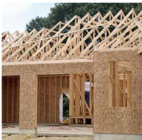
It is a structural product formed by chips or wood chips as a cross aligned to increase strength and rigidity higher layers. These chips are mixed with adhesives and chemicals by a heat press pressure likewise provides better insulation, high absorption, high stability, resistance to moisture and is easy to work. It is made from renewable materials that are environmentally friendly and they are certified Forest Management.
